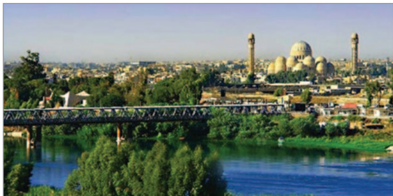
The Old Bridge, Mosul Nineveh Governorate
